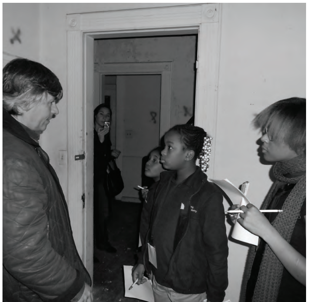
Pike International design manager Fernando Pastor gives Celentano Sentinel reporters a tour of the renovation project next to the school.
