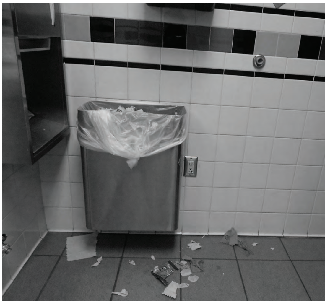
Overflowing trash on the second floor boys' bathroom floor.
